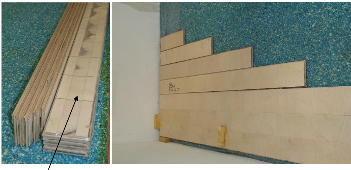
Backside of the Lumaflex panel – this side must be installed on the foam
