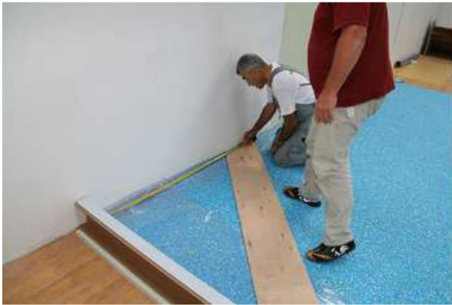
Installation of the first panel of Tarflex
