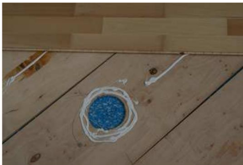
Before laying the top layer - Apply glue all around the recess you have created
