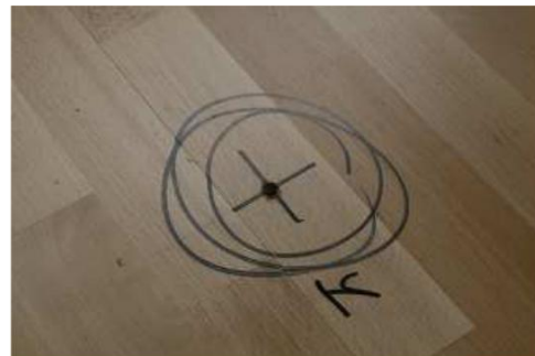
After having laid the top layer - locate the center of the anchor
