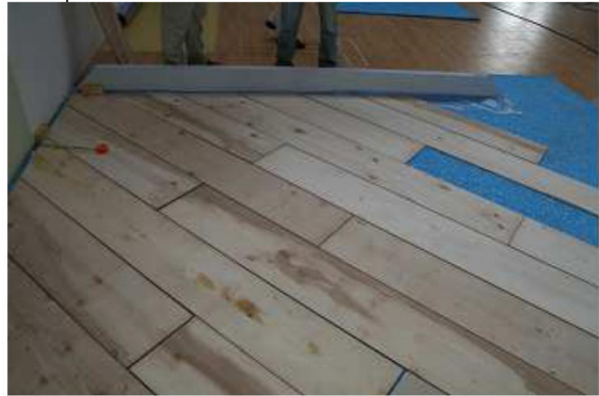
Special recommendation: always lay a complete panel board between two half panels
